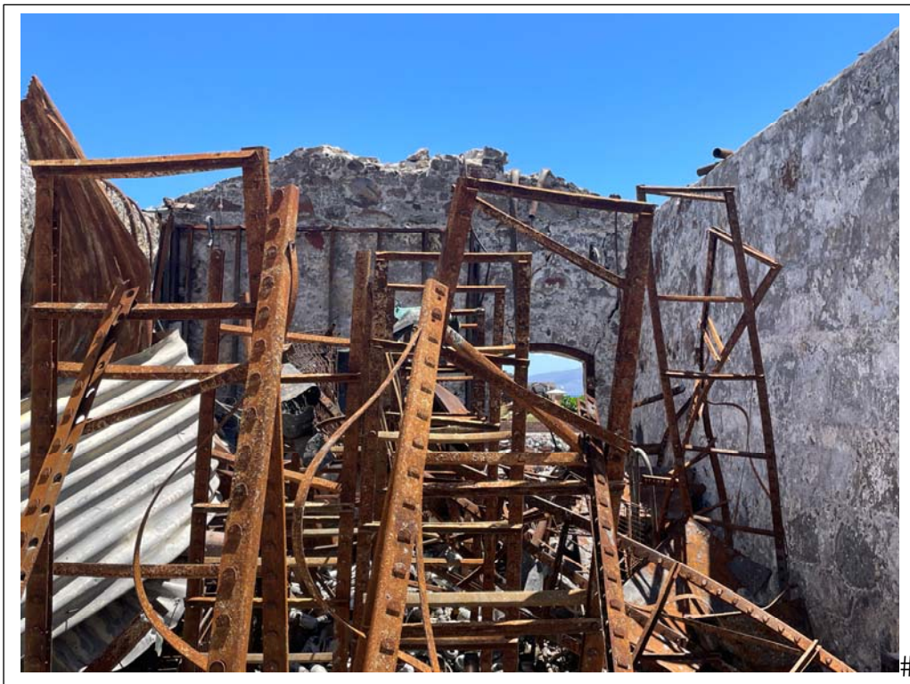
Interior of the “Spring House” (Photo KIP_7854, June 22, 2024).
